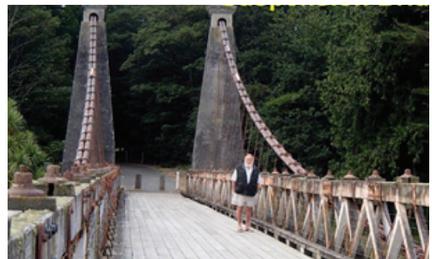
The Clifden War Memorial suspension bridge is New Zealand's longest wooden bridge, spanning 111.5 metres above the once mighty Waiau River.
