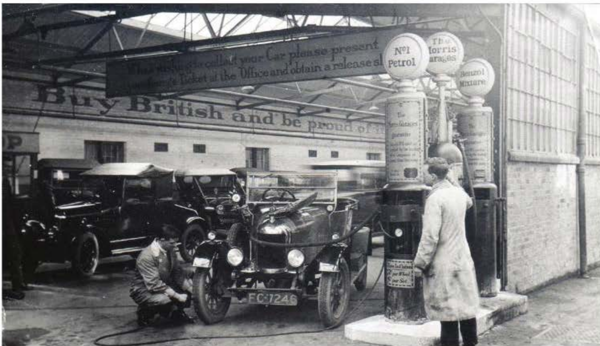
Clarendon Yard was rebuilt and turned into a covered area for storing/repairing cars. Petrol pumps were installed and used to fill the tanks of cars ready for collection. A sign on the back wall encourages people to buy British.
