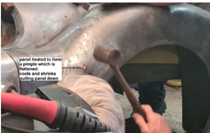
Heat shrinking a high spot
